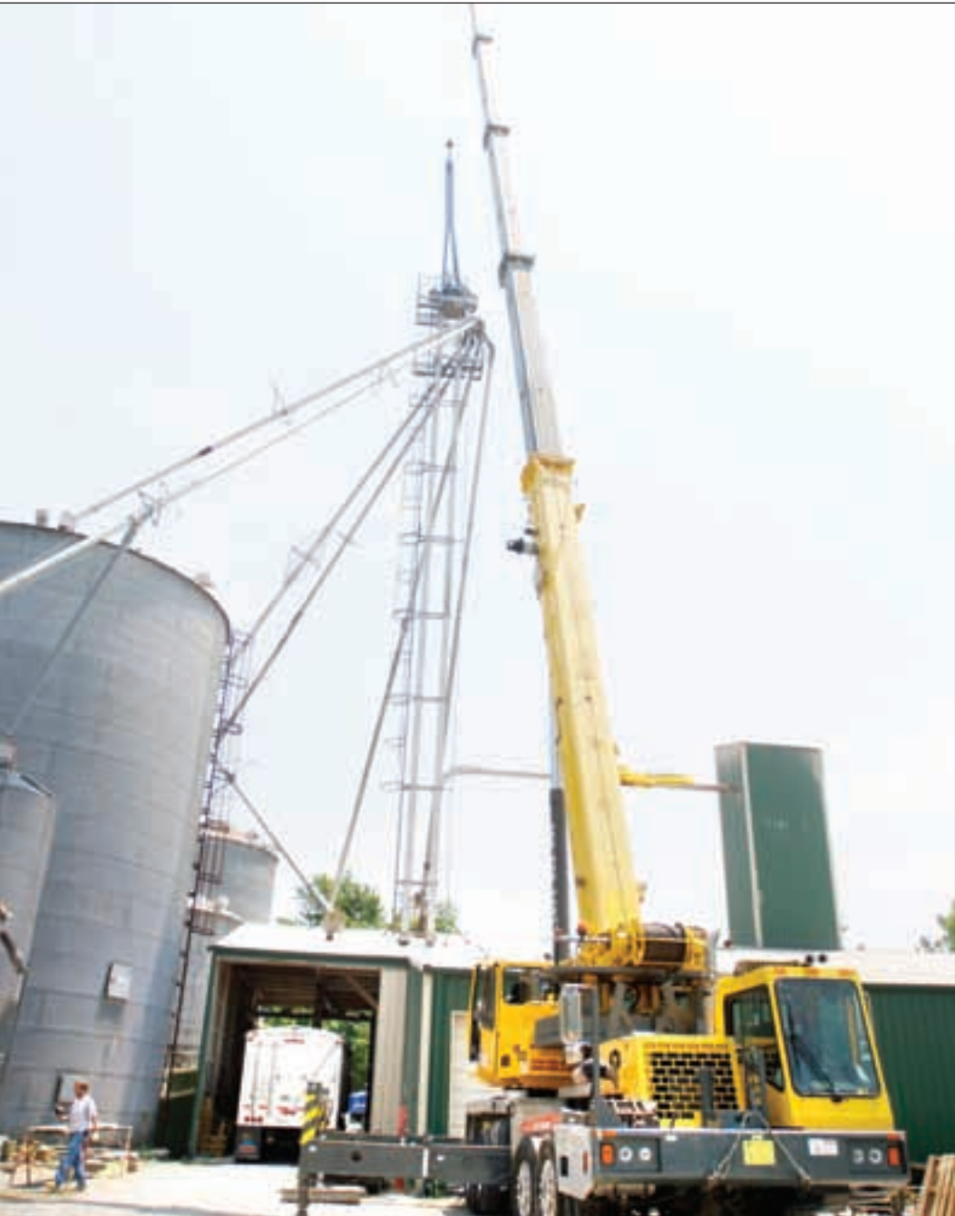
PHOTO BY JERRITT HOVEY-BROWN After a belt in the elevator leg that distributes corn broke recently at Marion Feed Mill, a crew from Hopkinsville was called to repair it. A crane that could reach 200 feet was needed and was brought from Clarksville, Tenn. Feed Mill Manager Keith Hart said the crew tried to repair the original belt, but it broke again. A new belt was purchased in Nashville and the crew installed it.
